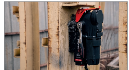
Working in out of positions
