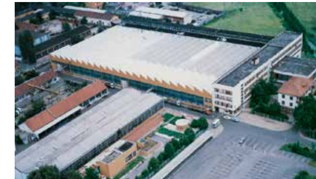
ZMM Nova Zagora production plant www.zmmnz.com
